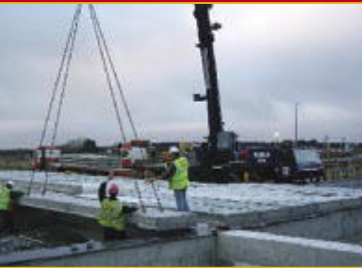
Placing Hollowcore
