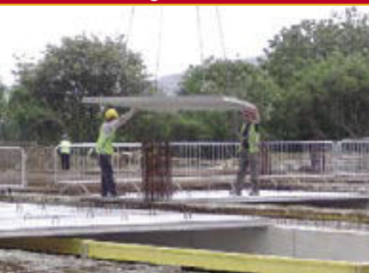
Placing Wideslab
